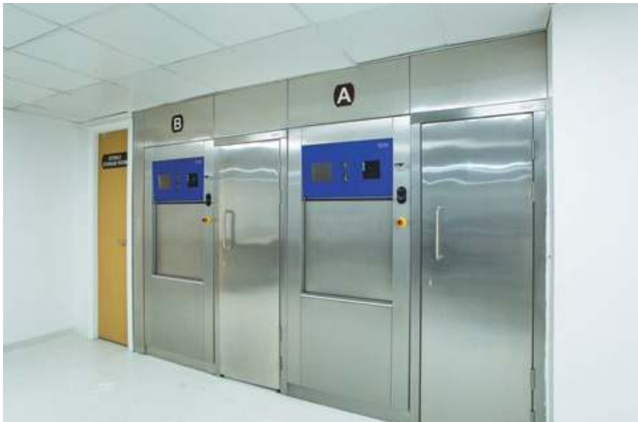
CSSD cladding with service door at SKS Hospital, Salem - India.
